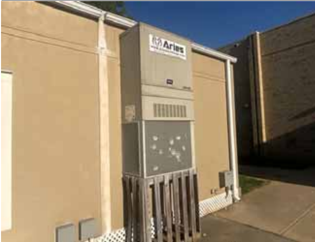
31 - WALL-MOUNTED HEAT PUMP
